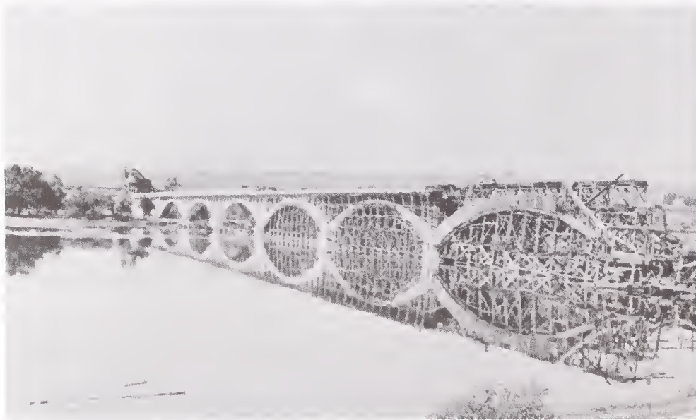
The partially completed bridge in 1920.
